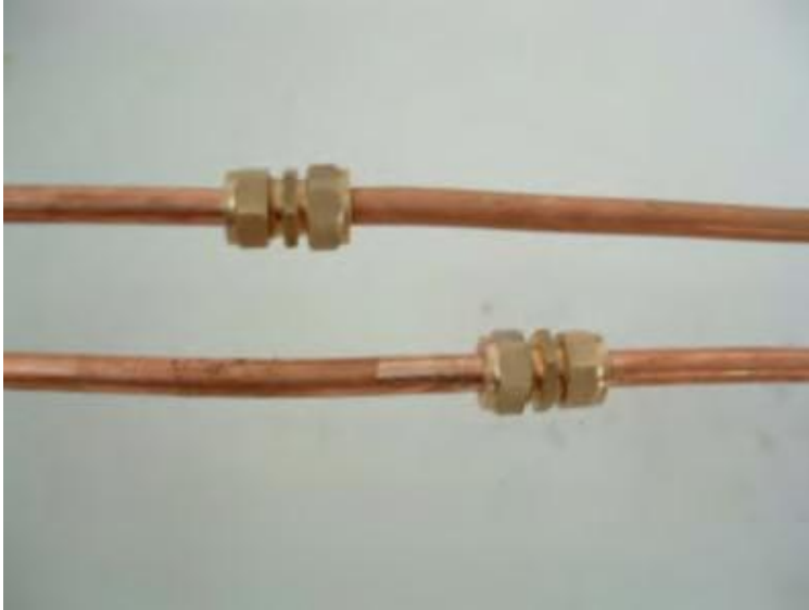
Joining copper pipe with unions
